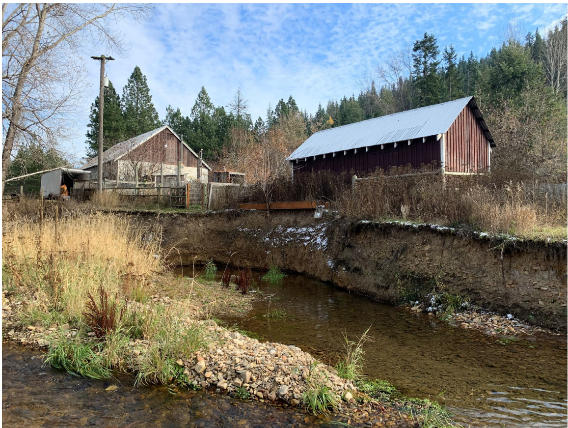
Photo 27: Pre-Construction. Left bank looking upstream. Downstream of property owner's structures. ( IMG_6840.jpg )
