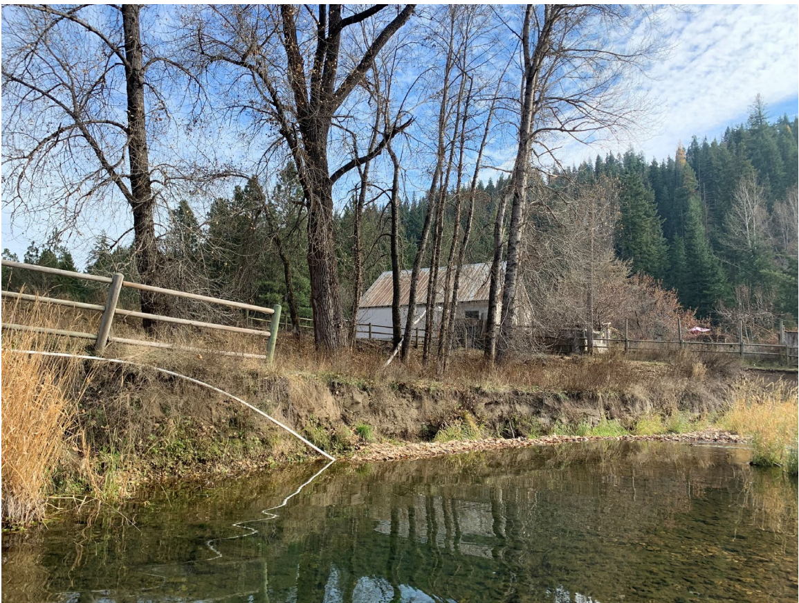
Photo 3: Pre-construction 10/31/2019. Left bank and stream channel, facing downstream. Upstream of property owner's structures. ( IMG_6838.jpg )
