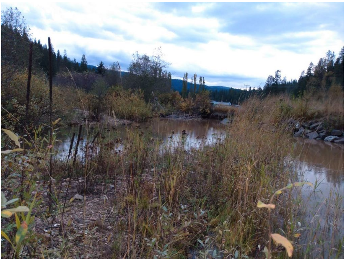
Photo 29: Pre-Construction. Stream channel, downstream of property owner's structures. Facing downstream. ( willow and flood plain before shot_Page_8.jpg )
