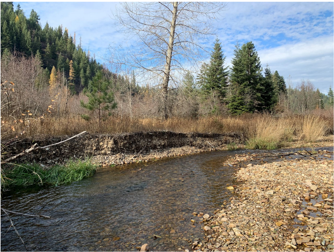
Photo 1: Pre-construction 10/31/2019. Right bank and stream channel, facing upstream. Near upstream end of project area. ( IMG_6810.jpg )
