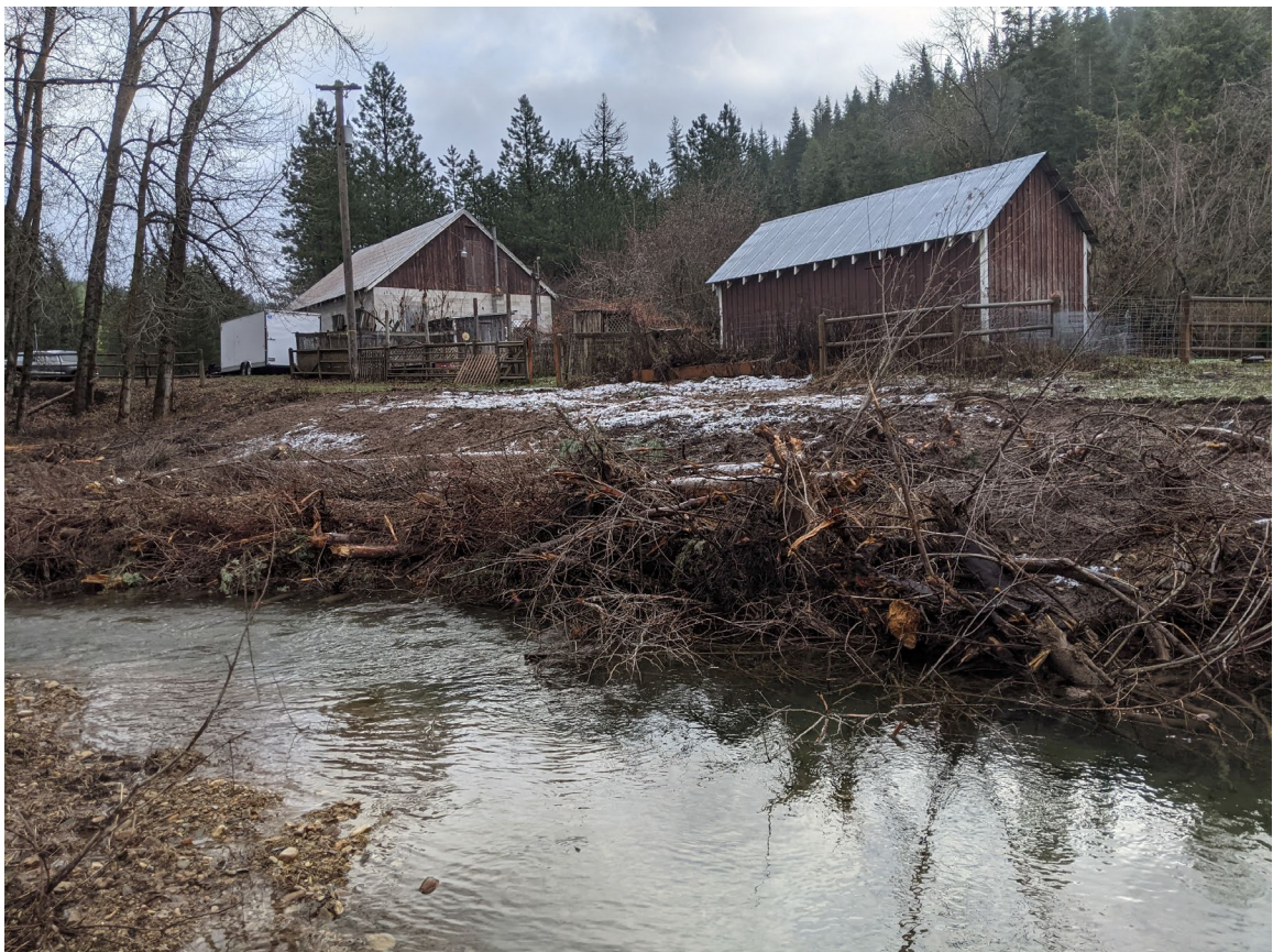
Photo 28: Post Construction. Left bank looking upstream. Downstream of property owner's structures. ( PXL_20201125_172841635.jpg )
