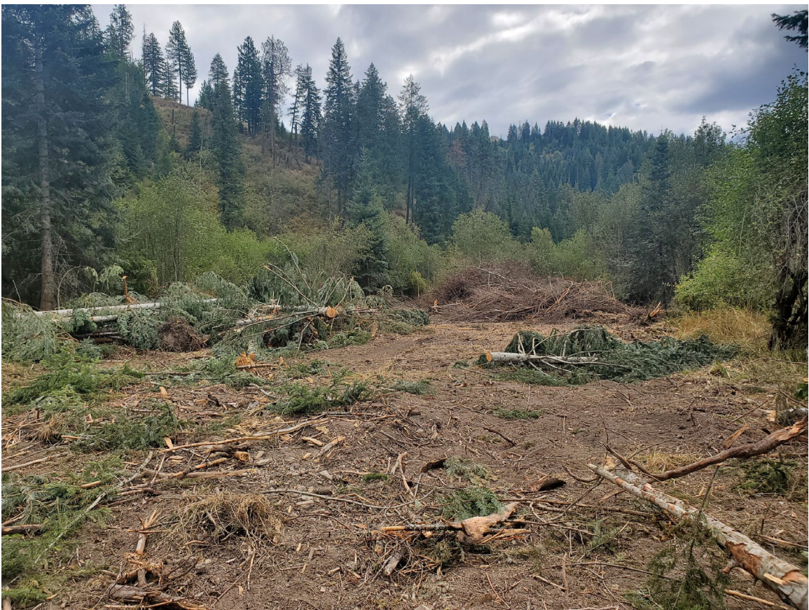
Photo 11: Construction. Staging area. ( Staging Area 1.jpg )
