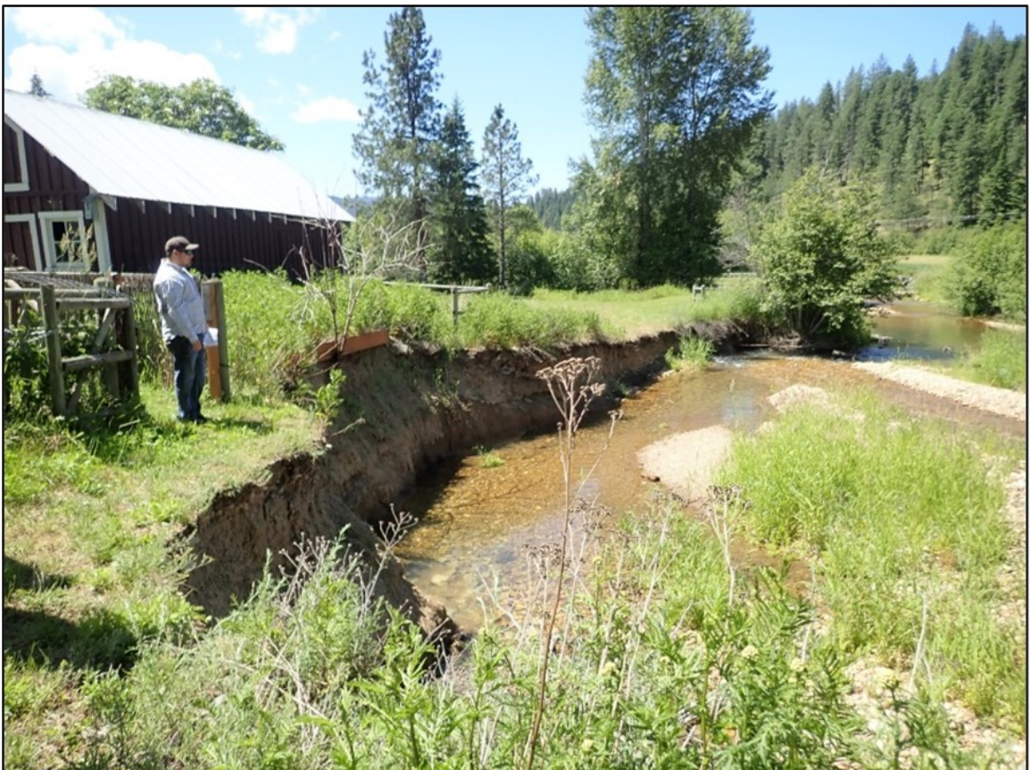
Photo 4: Pre-construction. Left bank, facing downstream. Near property owner's structures. ( Murphy Shed.jpg )
