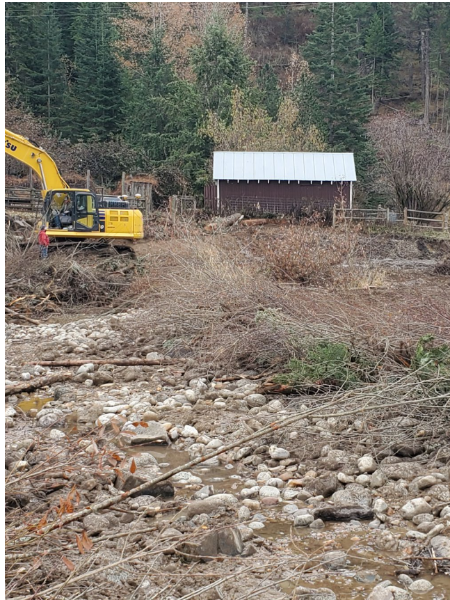
Photo 14: Construction. Floodplain treatment (right bank) with Vegetated Wood Matrix Type 1 and 2 installation (left bank). From right bank to left bank, near property owner's structures. ( Upstream looking at Mikes.jpg )
