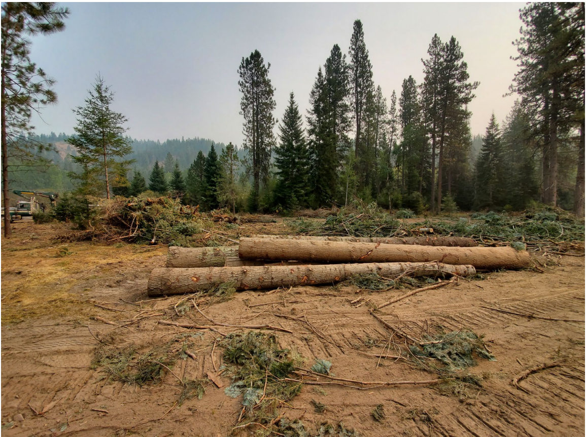
Photo 12: Construction. Staging area Category 3 wood. ( Cat 2 Staging Area.jpg )
