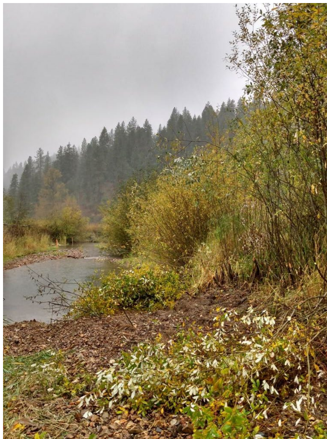
Photo 9: Construction. Willow harvesting. ( willow and flood plain before shot_Page_4.jpg )
