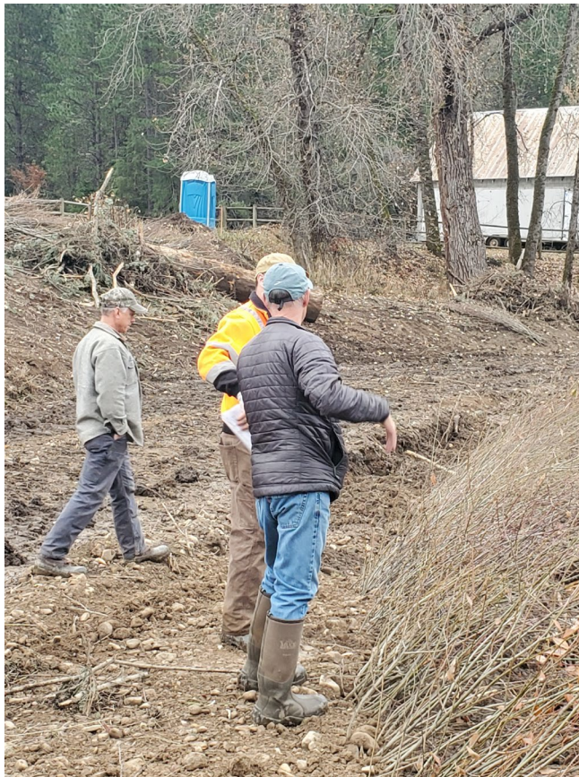
Photo 15: Construction. Inspection of Vegetated Wood Matrix Type 1 with partners . (1.jpg)
