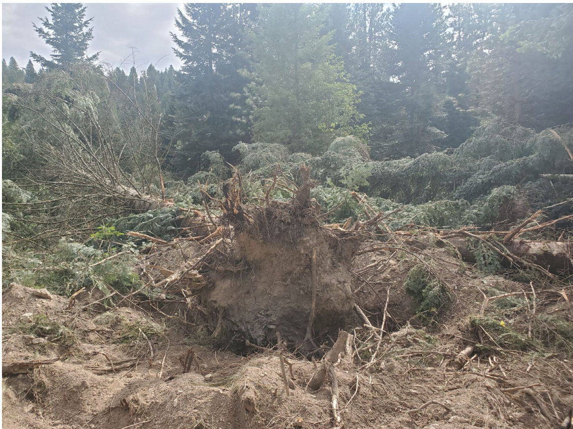
Photo 10: Construction. Collecting Category 1 wood. ( Cat 1 wood (a).jpg )
