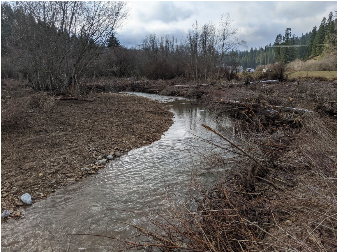
Photo 30: Post Construction. Stream channel, downstream of property owner's structures. Facing downstream. ( PXL_20201125_173122977.jpg )
